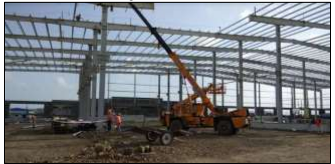
a. Assembling of inclined members (Site work of Nahar Industry Mandideep)
