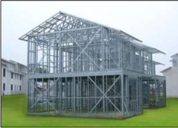
Fig. 1: Cold formed steel structure
