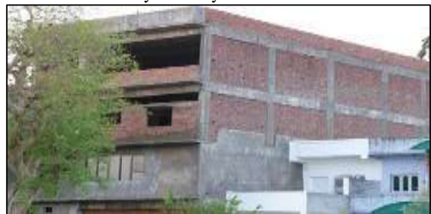
Fig. 2: RC frames with masonry infill walls
