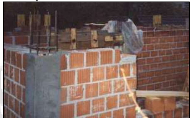
Fig. 1: Reinforced masonry wall
