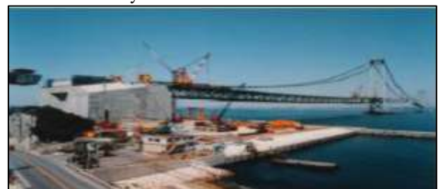
Fig. 1.3: Anchorage 4A of Akashi-Kaikyo Bridge
