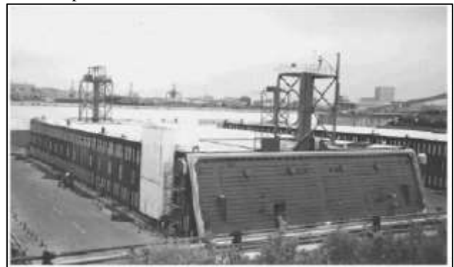
Fig. 1.8: Anchorage of Akashi-Kaikyo Bridge, Japan
