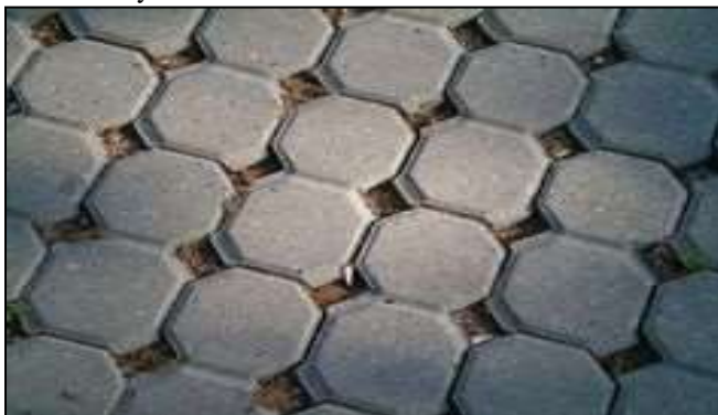
Fig.3: Pervious pavement using interlocking pavers
