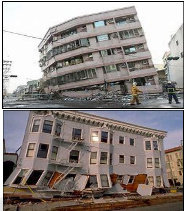
Fig. 1.1: Failure of Buildings Due to Earthquakes
