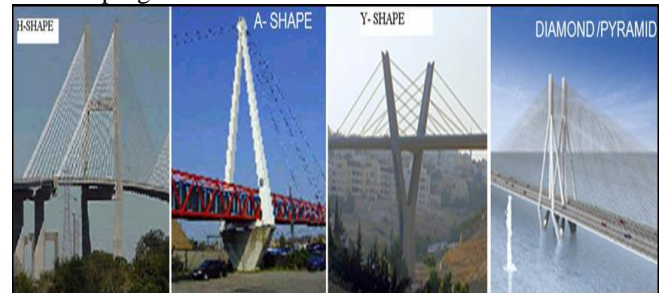
Fig. 1: Different tower/Pylons available for cable stayed bridge
