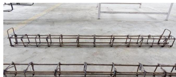
Fig. 6: Beam Reinforcement
