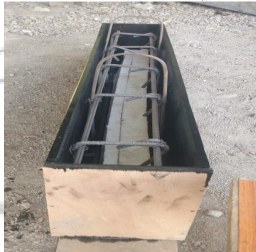
Fig. 3: Detail for mould with reinforcement and thermocol
