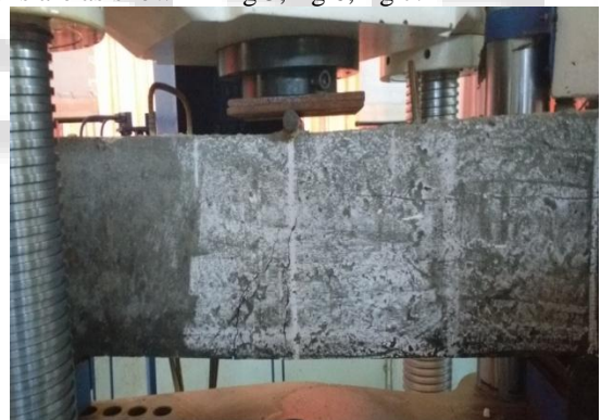
Fig. 5: crack pattern (control beam)
