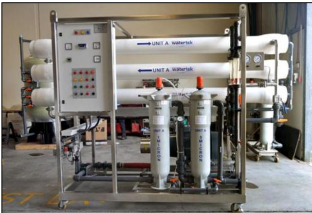
Fig. 2: Commercial RO Plant Sangamner RO Plant is under consideration for case study.
