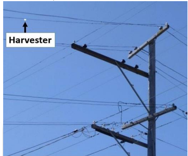
Fig. 1: Hypothetical energy harvester (to scale) attached to an overhead power distribution line
