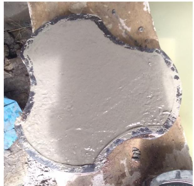
Fig. 4: manufacturing of paver block
