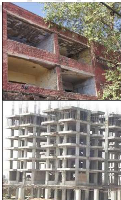
Fig. 3: load bearing structure & frame structure
