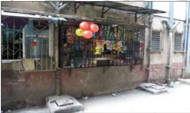
Fig. 5: Residential building is used as commercial building
