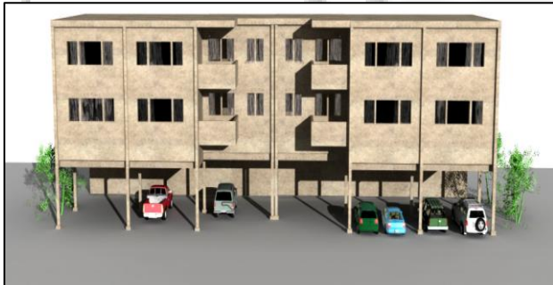
Fig. 1: Open Ground Storey
