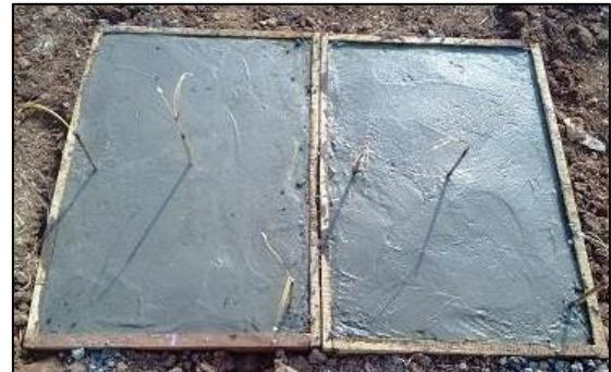
Fig. 1.11: Finished Surface of Slabs
