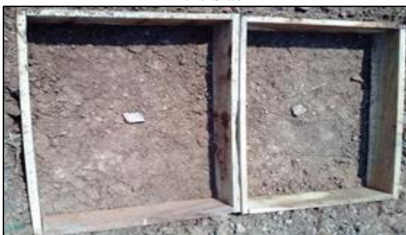
Fig. 1.9: Excavated Ground Surface
