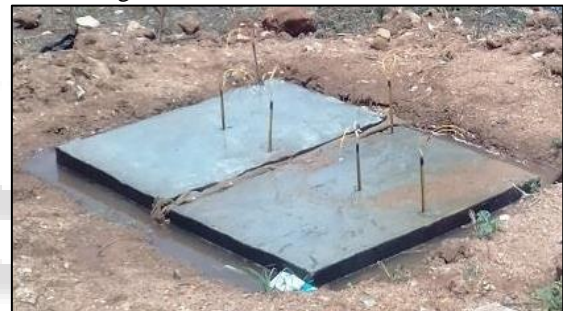
Fig. 1.12: Curing of Slabs
