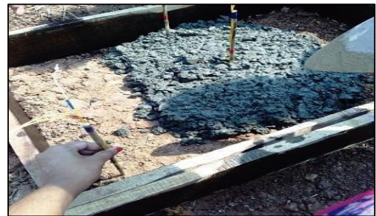
Fig. 1.10: Placing Of Thermocouples at Interior, Edge and Corner
