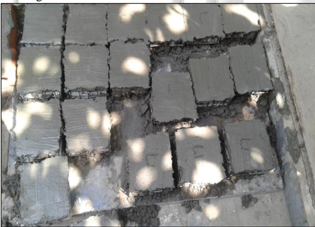
Fig. 3: Plastering of EPS Panels
