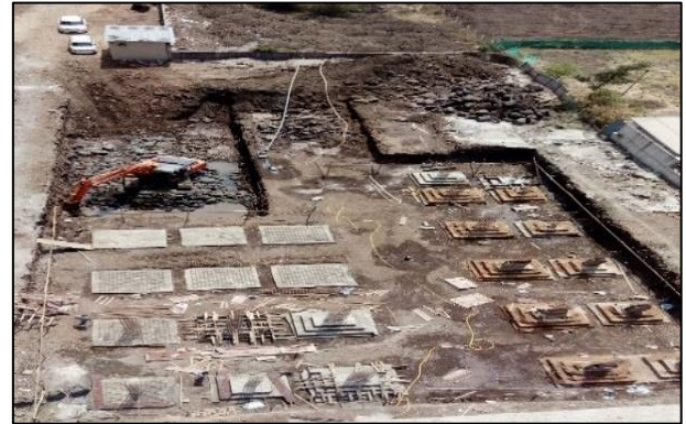
Fig. 8: 1 st phase Completed
