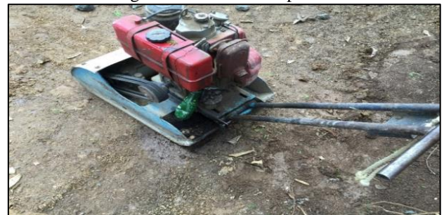
Fig. 10: Vibrator Dressing of Base Course
