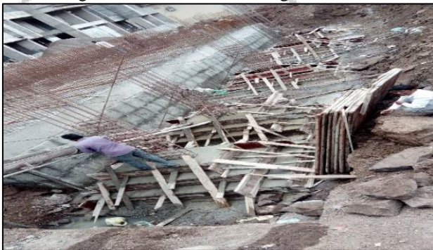
Fig. 5: Casting of Footing and Column
