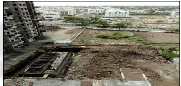
Fig. 9: Part Work Completed
