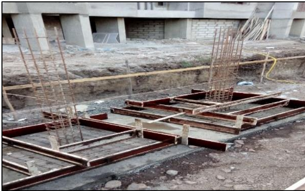
Fig. 4: Formwork For Footing & Column
