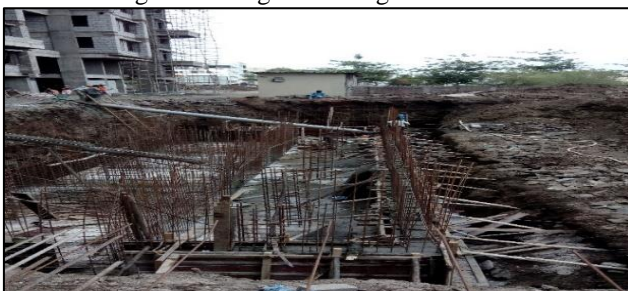
Fig. 6: Casting Work of Second Phase
