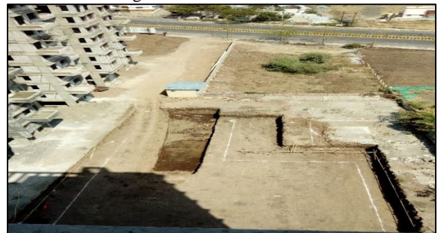
Fig. 2: Excavation Work For Footing
