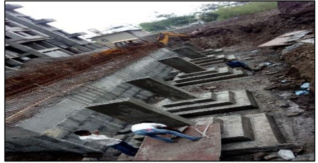
Fig. 7: Post Concreting Work
