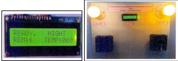
Fig. 4.2: When 6 people enters room, 2 light and 2 Fan starts
