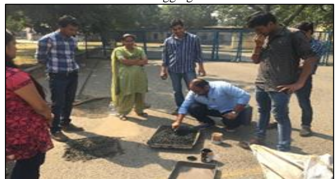
Fig. 15: potholes in CSIR-CRRI Campus
