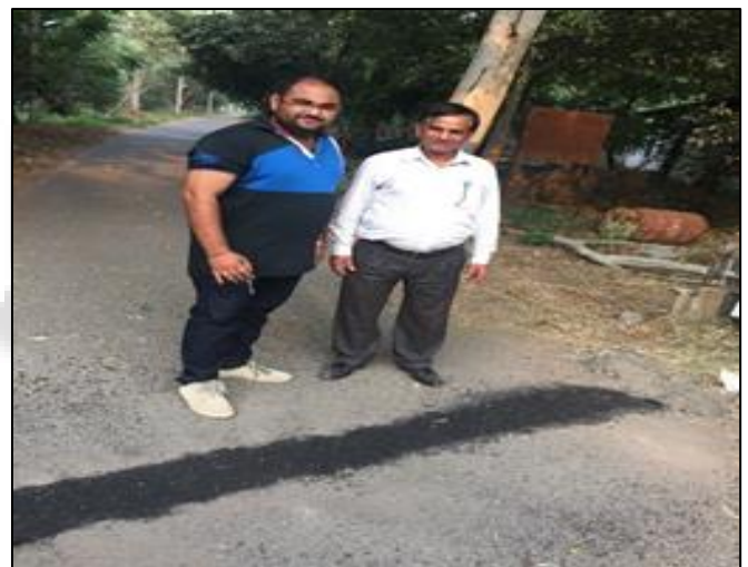
Fig. 14: Pothole repair in NTPC badarpur with coal mix waste aggregate
