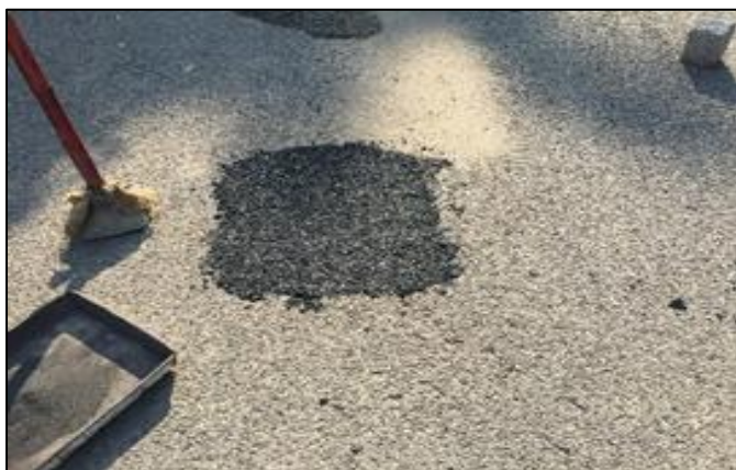
Fig. 16: potholes repair in CSIR-CRRI Campus with coal mix waste aggregate
