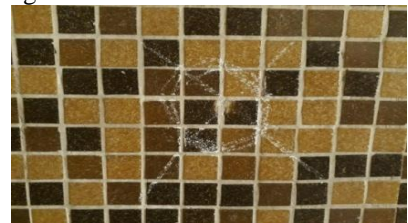
Fig. 5: Field test applying point
