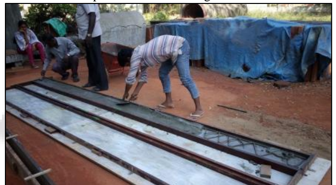
Fig. 5: Middle layer casting with reinforcement
