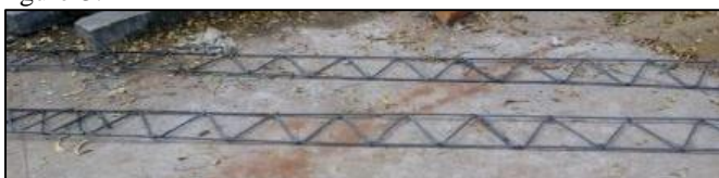
Fig. 3: shear reinforcement of rectangular joist
