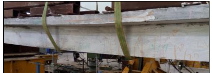
Fig. 8: Crack pattern above 6-t loadings
