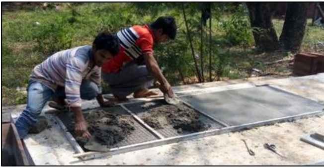
Fig. 6: Precasting of ferrocement planks
