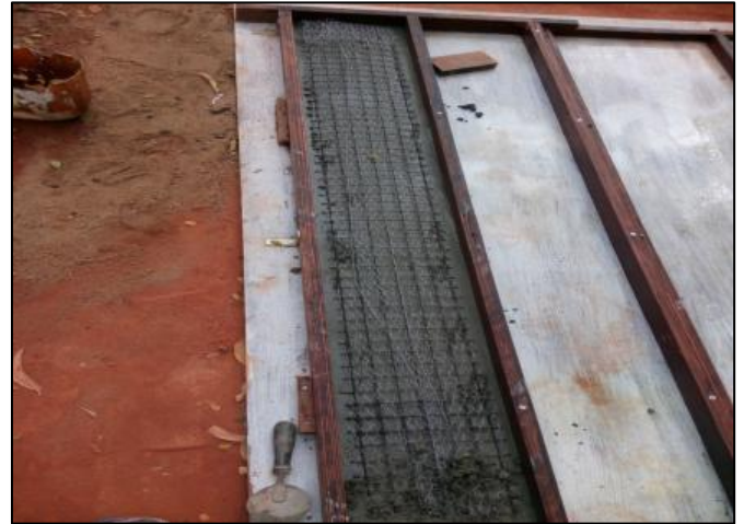
Fig. 4: Layer by layer casting of rectangular joist
