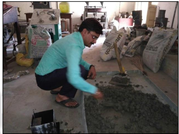
Fig. 1: Mixing of Concrete
