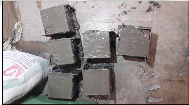
Fig. 2: Casting of Concrete in Moulds
