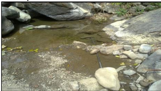
Fig. 8: A pipe is fixed into the pool of a stream and supported by stones from moving astray
