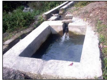
Fig. 3: A storage tank along the stream
