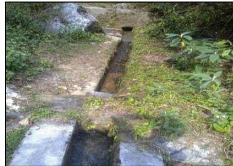
Fig. 4: A narrow channel connects the stream to the tank
