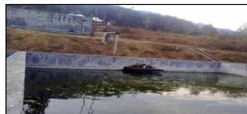
Fig. 6: Water flows inside one of the reservoir tanks for detention
