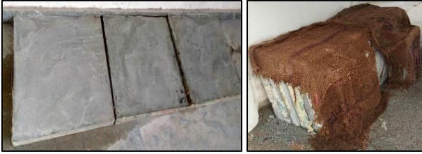
Fig. 3: Demoulding (a) and curing with gunny bags(b).
