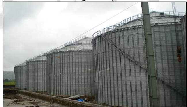
Fig. 2: Silos with corrugated sheet and vertical stiffener
