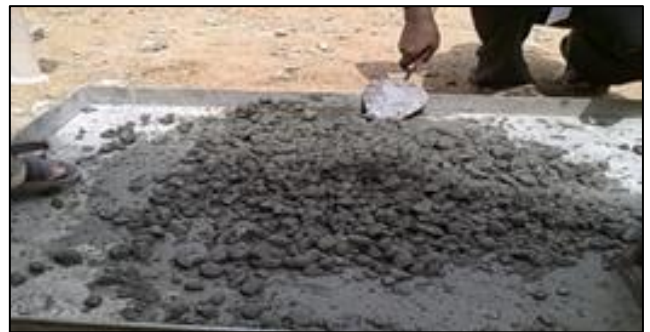
Fig. 1: Mixing of Concrete
