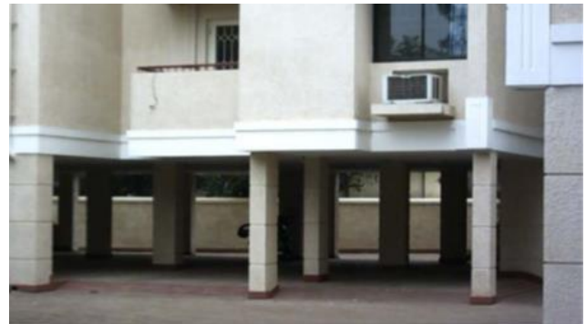
Fig. 1: Typical Soft Storey in India
