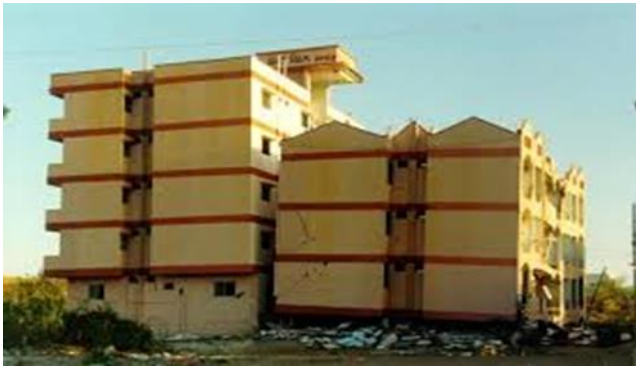
Fig. 4: Typical Soft Storey Failure in Bhuj Earthquake.
