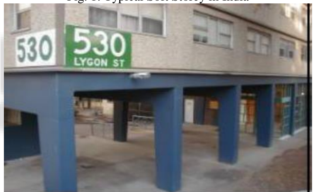
Fig. 2: Typical Soft Storey in Australia
