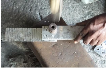
Fig. 6: Preparation for Riveted Joint
