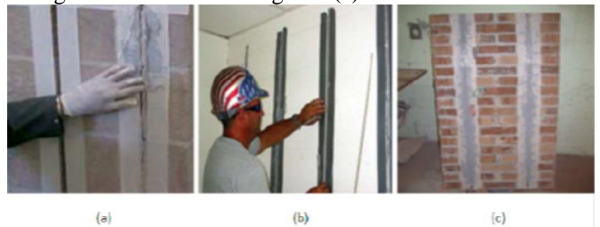
Fig. 6: Masonry wall is strengthened in vertical direction using NSM FRP reinforcement
