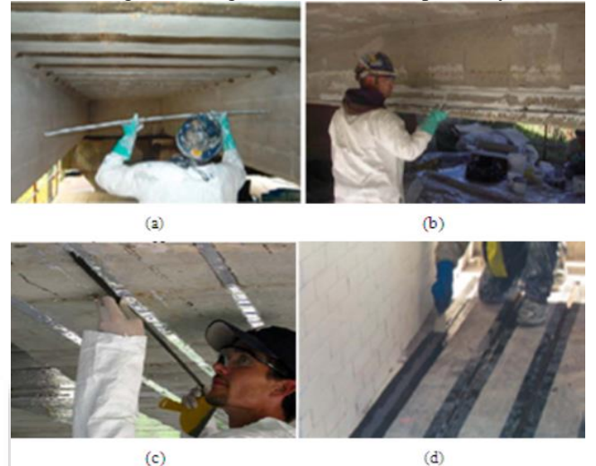
Fig. 4: RC elements strengthened using NSM FRP
