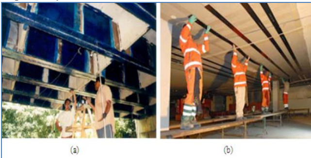
Fig. 2: Field applications of FRP using EBR method
