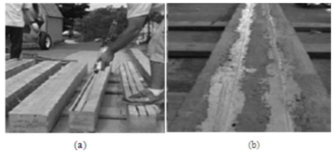
Fig. 3: Strengthen using NSM Technique.
