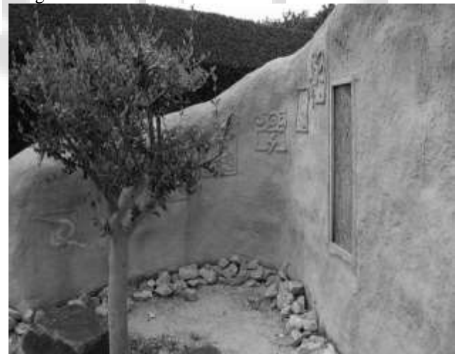
Fig. 13: Boundary wall made with Mud.
