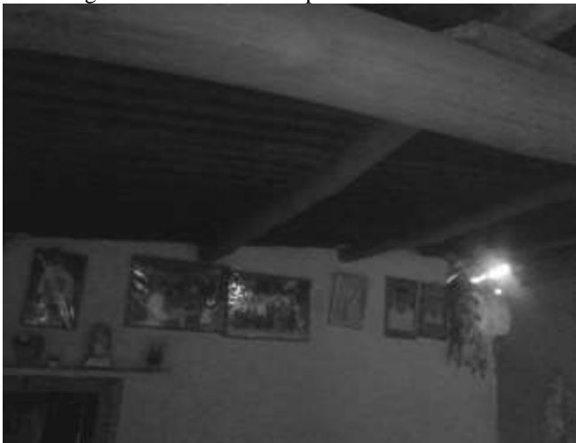
Fig. 10: Rafters and Purlins of tin-roof of a mud house in Bercha.
