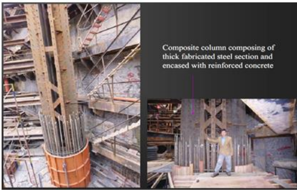
Fig. 2: Typical encased composite column section
