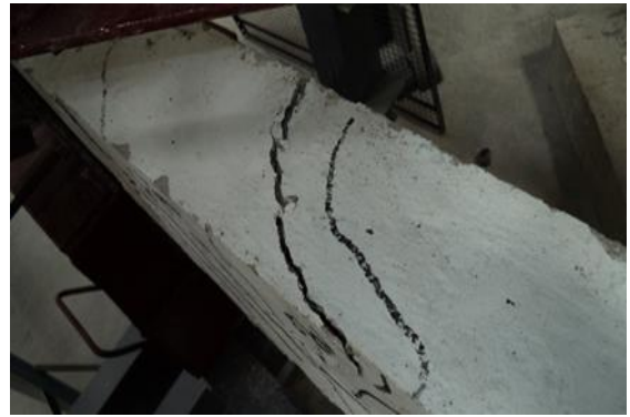
Fig. 9: Failure pattern of Conventional beam
