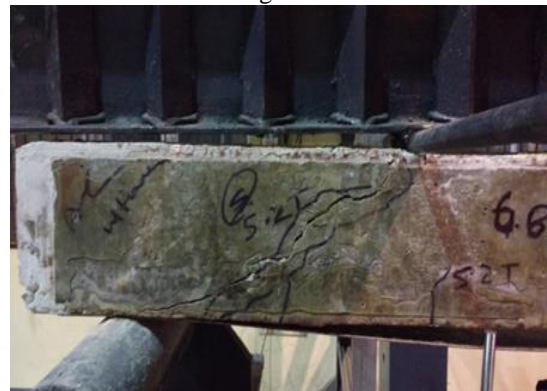
Fig. 12: Typical failure of RC strengthened beam with continuous steel sheet (2 mm) at bottom and side faces
