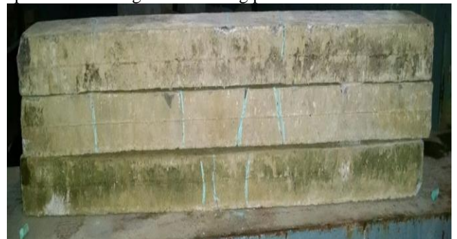
Fig 7: Showing Cracking And Failure Pattern
