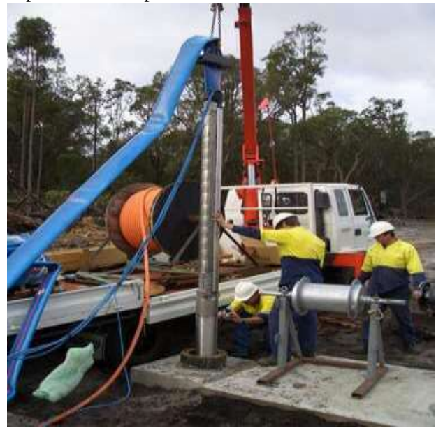
Fig. 5: Hydraulic operated submersible motor lifting machine.
