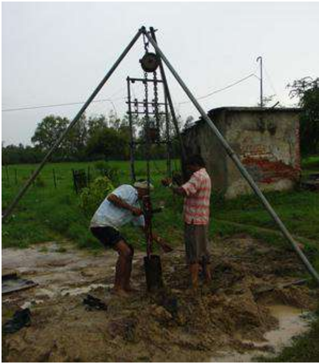
Fig. 4: Chain pulley block mechanism.
