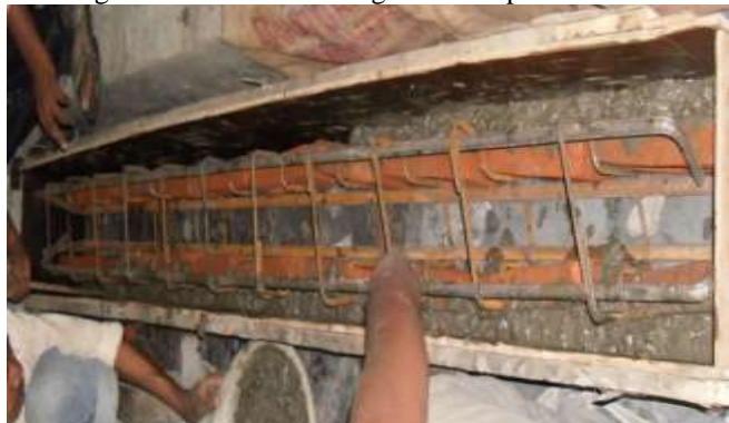
Fig. 4: Casting of Beam
