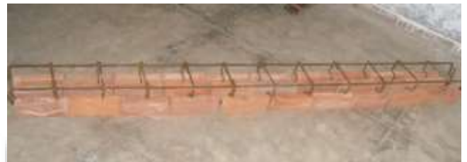
Fig. 2: Arrangement of Bricks with Reinforcement Cage
