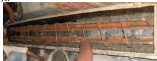
Fig. 4 Casting of Beam
