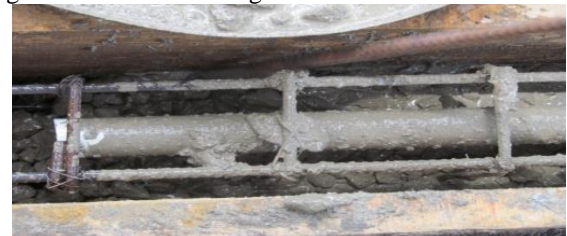
Fig. 4: Casting of hollow beam
