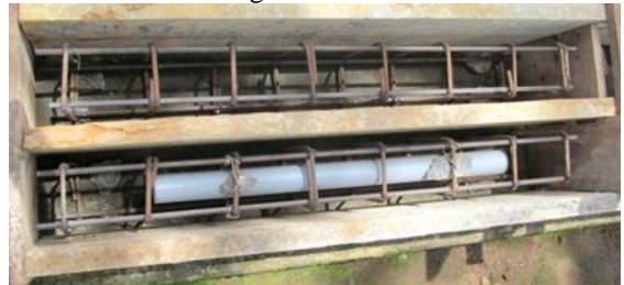
Fig. 3: Reinforcement cage inserted inside the formwork
