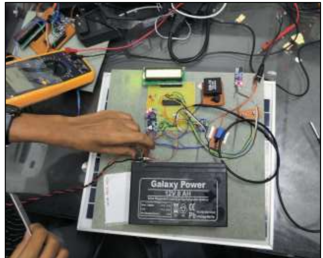
Fig. 2: Solar EV Charging Station
