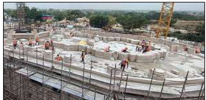
Fig. 3: construction of ram temple
