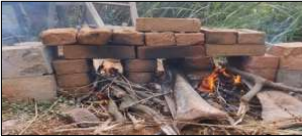
Fig. 10: Burning of Bricks
