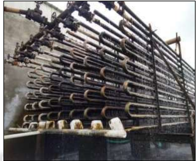
Fig. 3: Construction of Atmospheric Condenser
