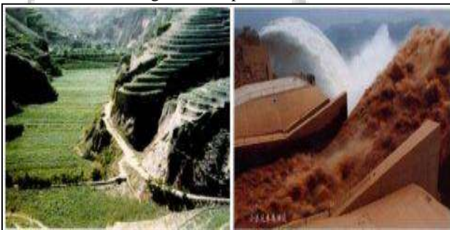
Fig. 3: Sediment Removal, reduction, and flushing
