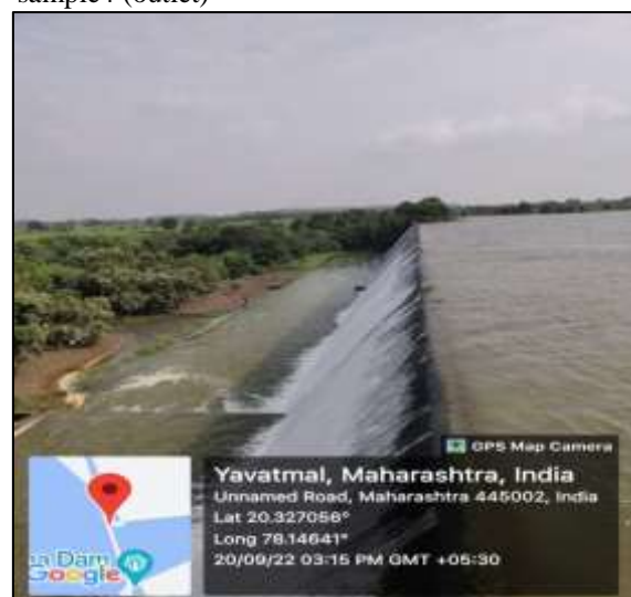
Fig. 1: Large view of Nilona dam
