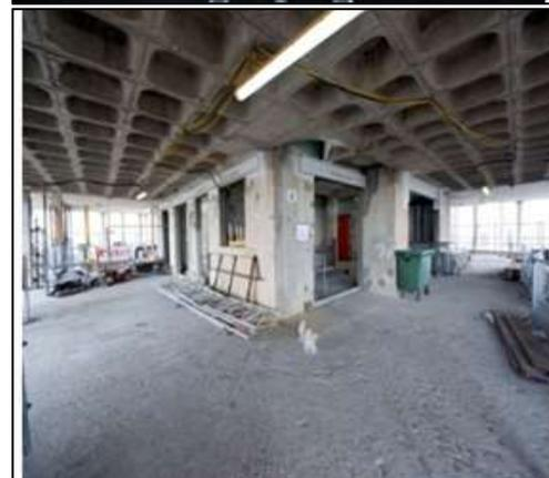
Fig. 1: Typical examples of waffle slab
