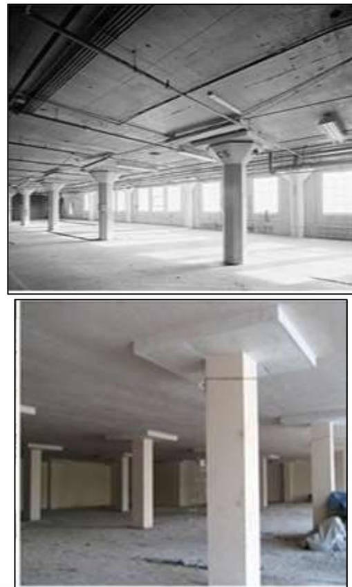
Fig. 3: Typical examples of flat slab
