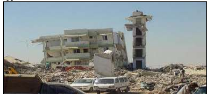
Fig. 1: collapse in bhuj (2001)
