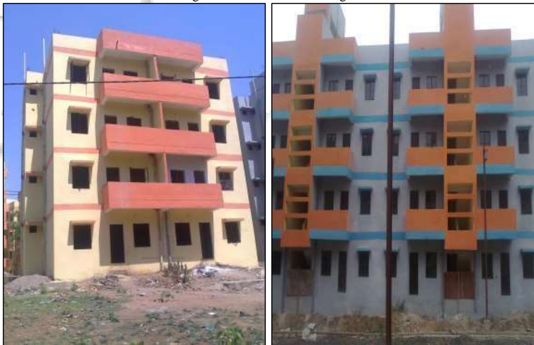
Fig. 4: Constructed Dwellers Unit under Jnnurm ( Jablpur)
