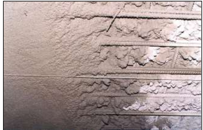
Fig. 1: concreting of fire damaged slab
