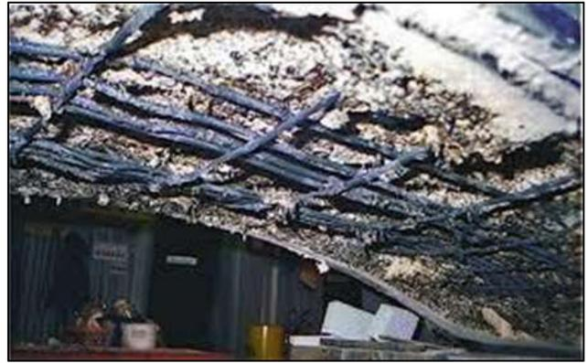
Fig. 1.4: Spalling of Concrete due to Fire
