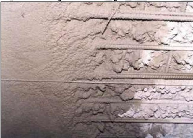
Fig. 1.2: Concreting of Fire Damaged Slab
