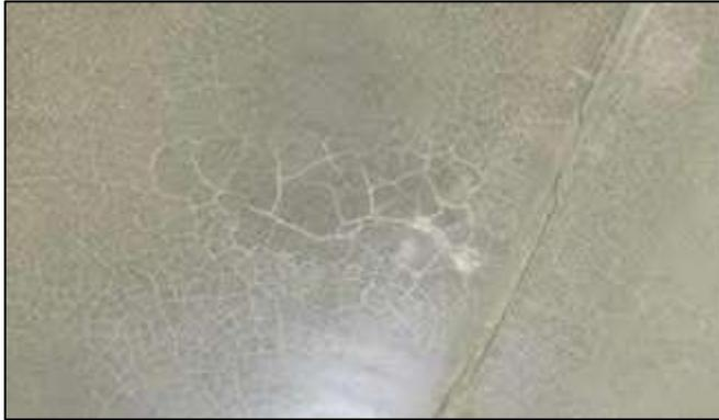
Fig. 1.5: Delamination of Concrete 1.5: Tests to be conducted on the RCC structure.
