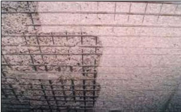
Fig1.1: Fire Damaged Slab
