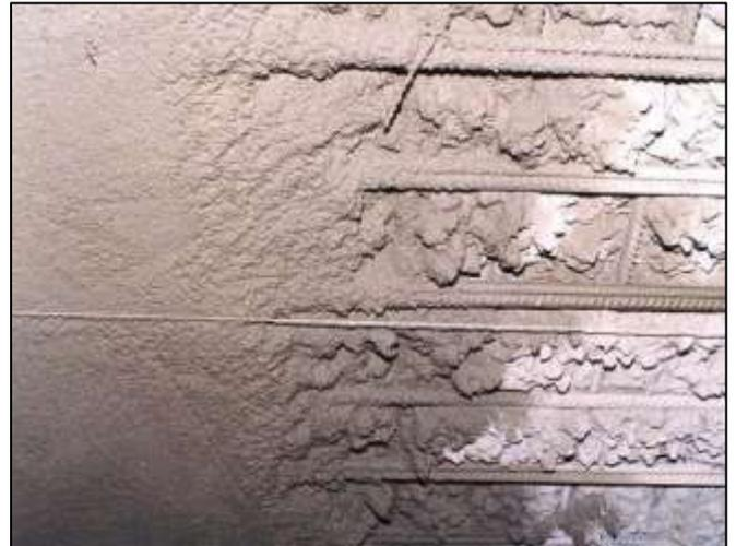
Fig 1.2: Concreting of Fire Damaged Slab
