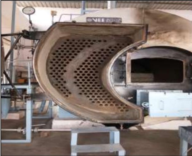
Fig. 5: Biomass Boiler
